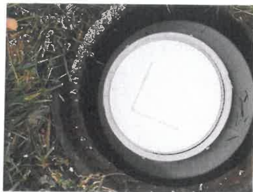
Picture inside the metal box cover
