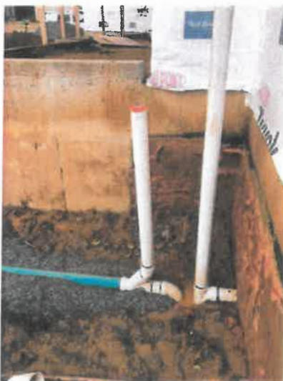
Typical Vent-Trap Configuration
