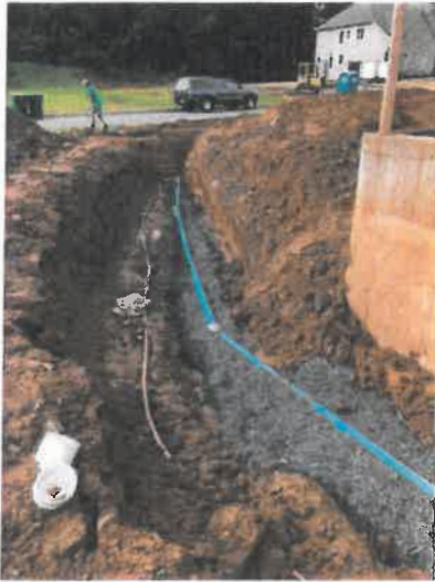
Typical SDR-26 Pipe Installation
