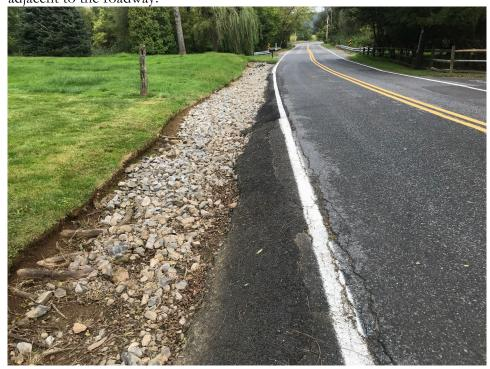
Shows no shoulders with "alligator" cracking repair along the roadway near Courtney Street.
