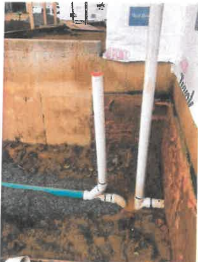
Typical Vent-Trap Configuration
