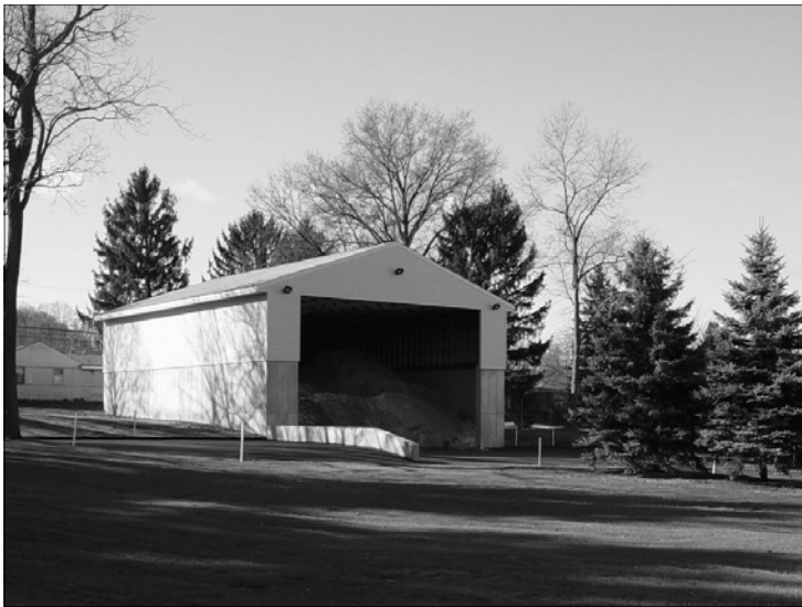
The newly built Township salt and anti-skid storage building
